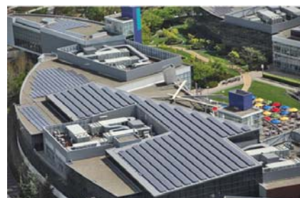
1.6MWp PV system at Google HQ
