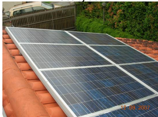
Retrofitted – PV modules are mounted on the existing roof tiles.
