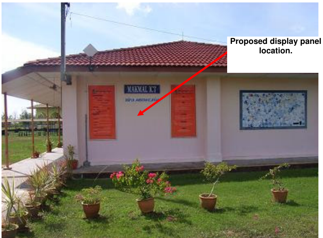
Side view of Makmal ICT SMK Lutong (PV array to be installed at Makmal ICT roof). APVSPs are required to measure and ensure that the roof space is sufficient to locate the PV array.
